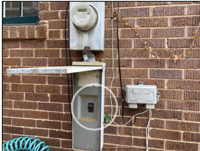
77. main electrical disconnect
