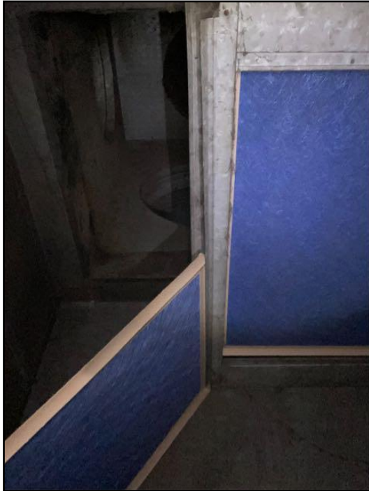
85. Air filter location at furnace
