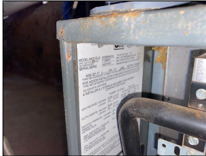
84. Furnace data plate
