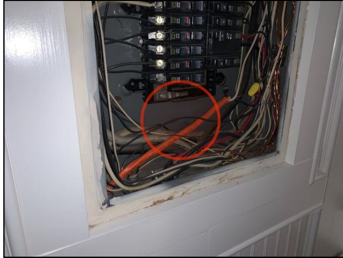
52. Excessive sheathing length
