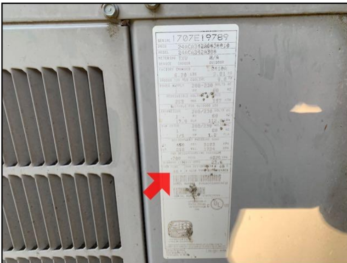
87. AC data plate calls for max 40 amp breaker
