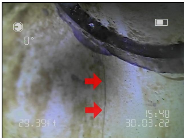
9. Cracking at 29.39'.
