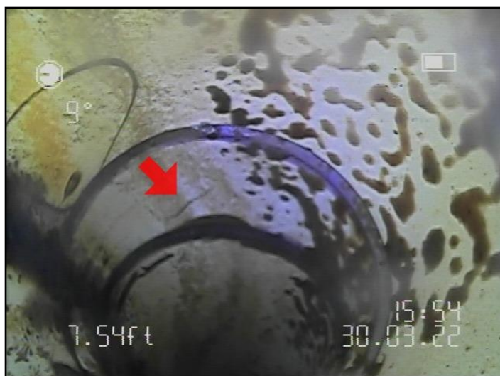
11. Cracking at 7.54'.
