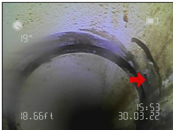
10. Cracking at 18.66'.
