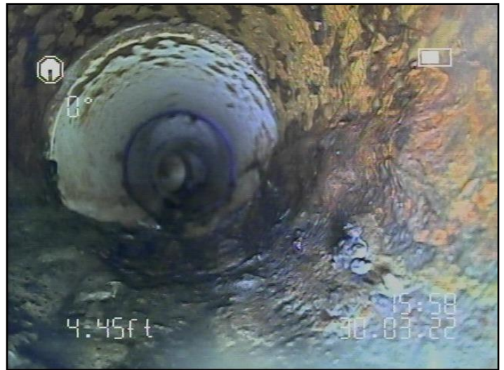
15. Cast Iron to PVC at 4.45'.
