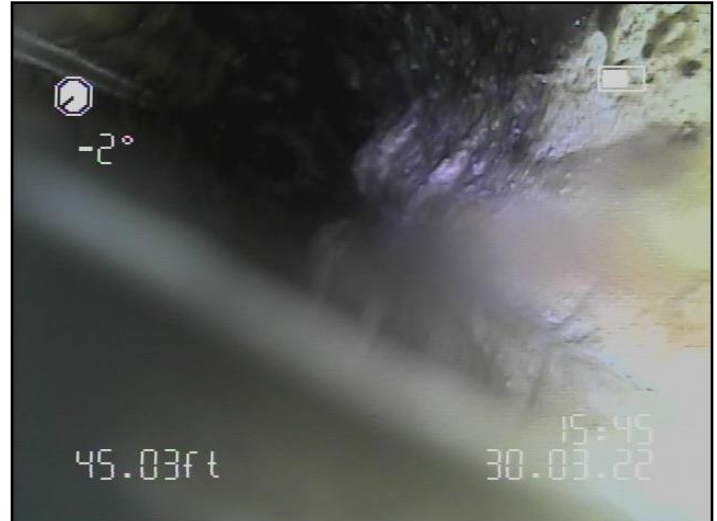
7. Belly/Settling in pipe at 45.03'.
