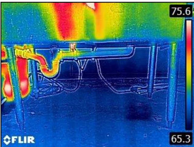
131. Laundry Area: No issues
