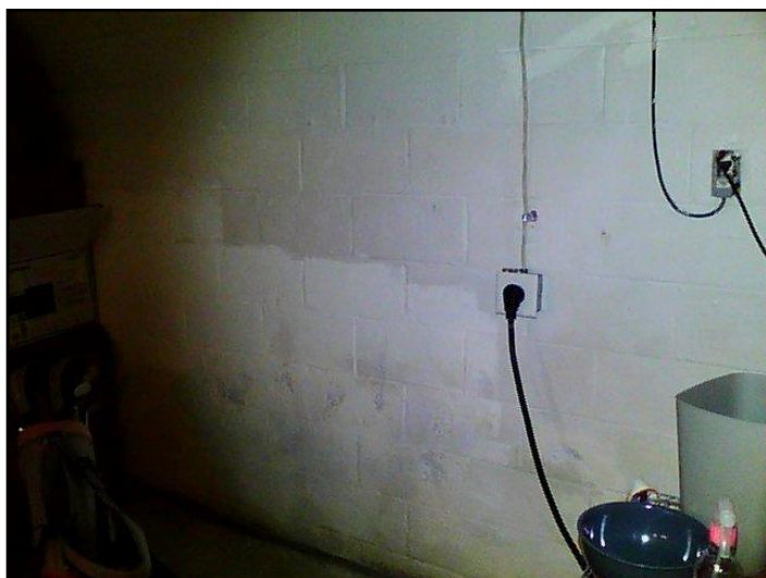
136. Below Grade Foundation Walls: No issues
