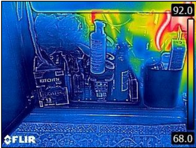
97. Kitchen: No issues
