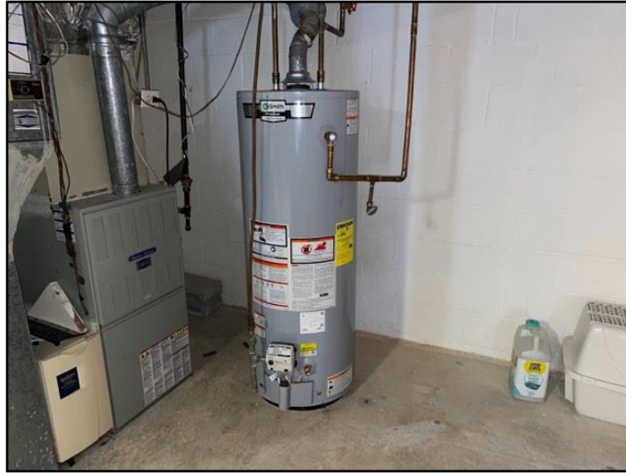
65. Conventional (Tank) Gas Fuel - 8-12 Years...
