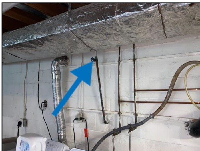
64. Front of the basement
