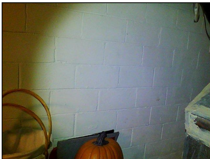
134. Below Grade Foundation Walls: No issues
