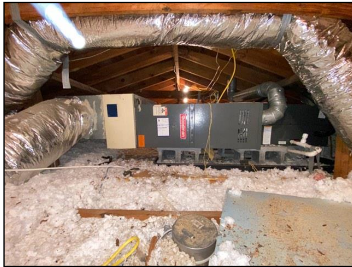
38. Mid-Efficiency Gas Furnace - 18-25 Year Lif...
