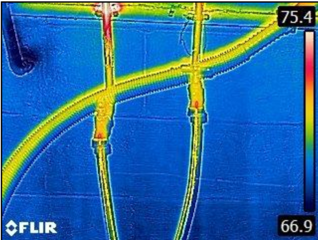
129. Laundry Area: No issues
