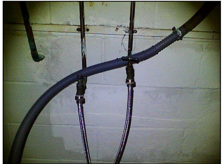
130. Laundry Area: No issues
