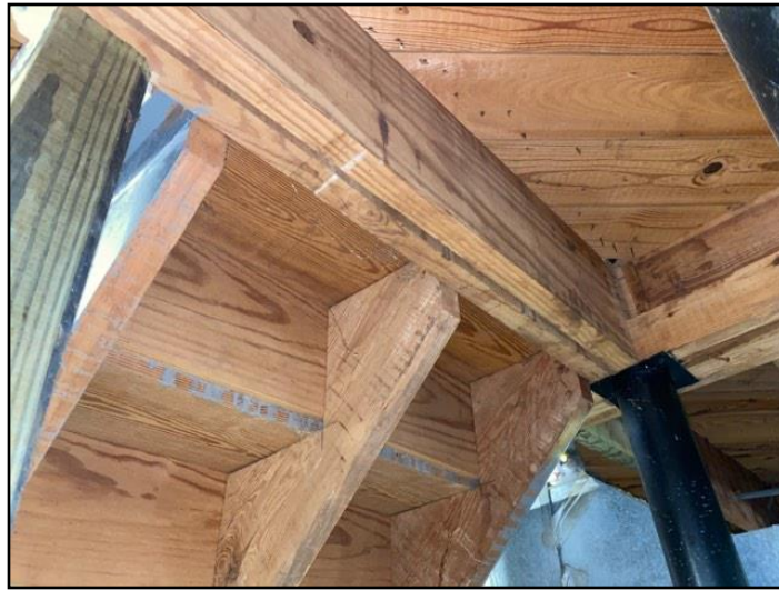
83. Poorly supported
