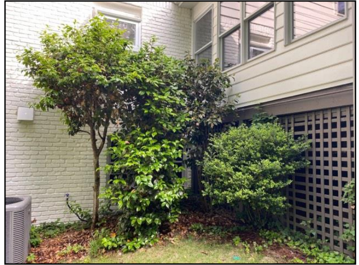
21. Trees or Shrubs too close to building
