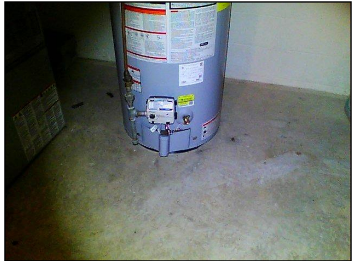
126. Plumbing Fixture/Penetration: No issues
