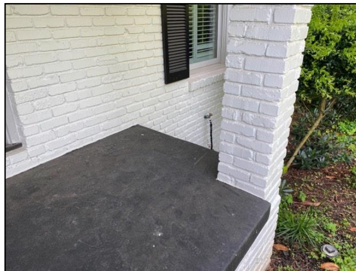
14. Guardrail Missing
