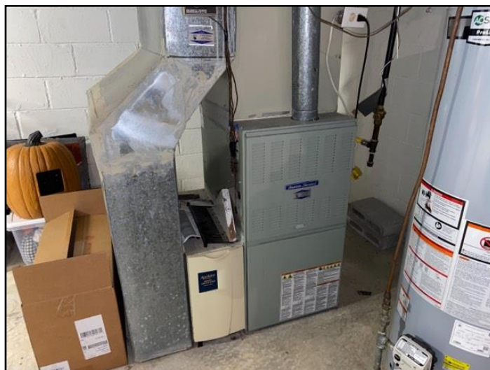
39. Mid-Efficiency Gas Furnace - 18-25 Year Lif...
