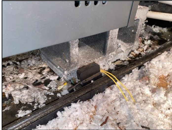
47. Debris in auxiliary pan
