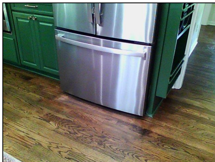
96. Kitchen: No issues
