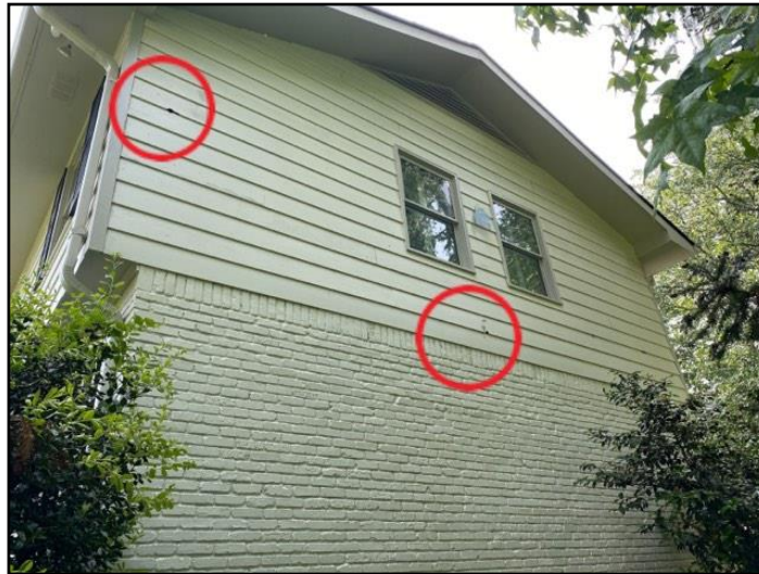
10. Rot/Insect damage
