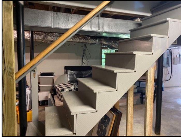
81. Guardrail Missing
