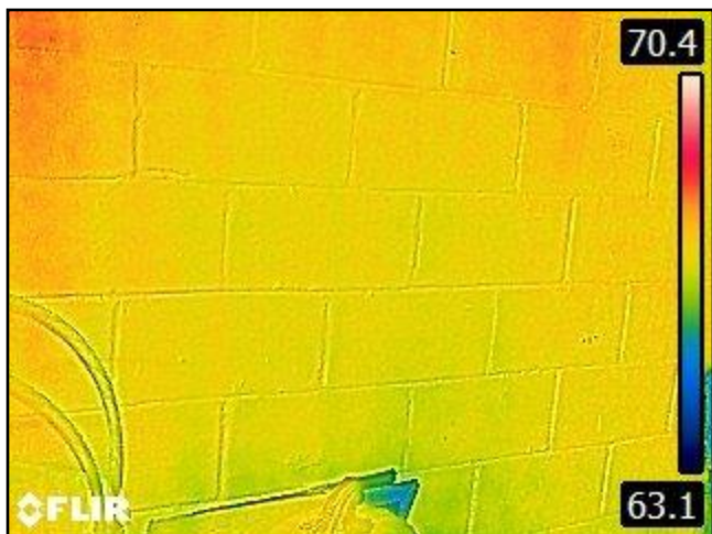
133. Below Grade Foundation Walls: No issues
