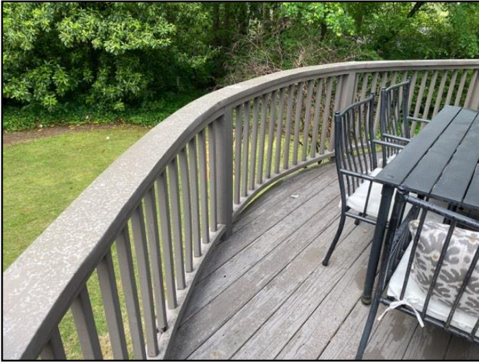
15. Loose/weak Guardrail
