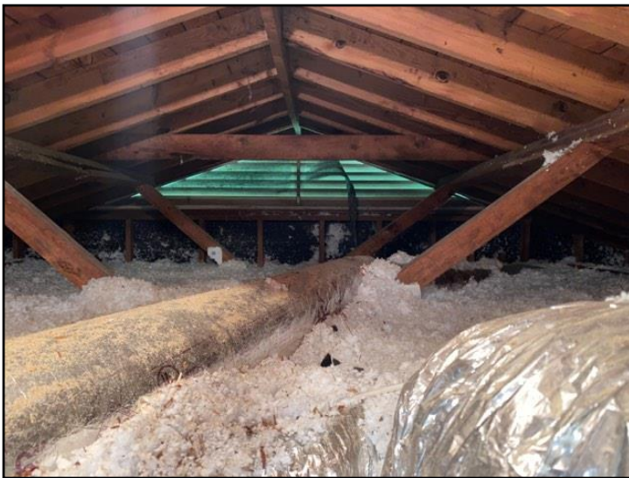
52. By entering attic, but access was limited
