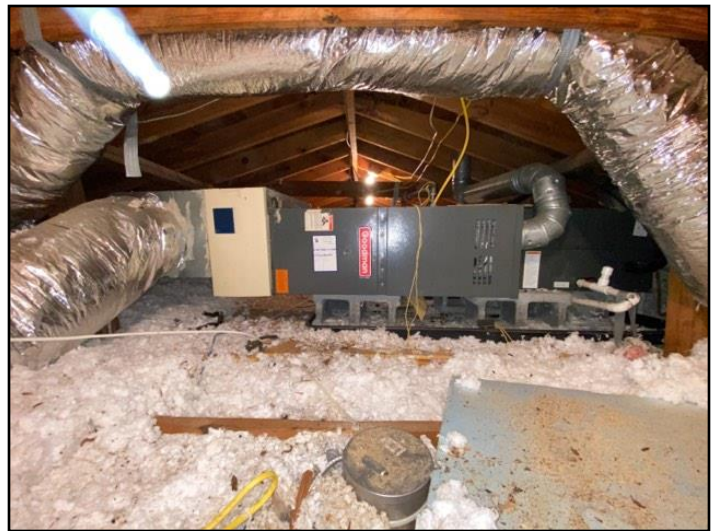
53. By entering attic, but access was limited
