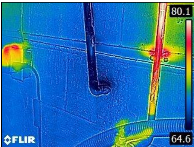
123. Plumbing Fixture/Penetration: No issues
