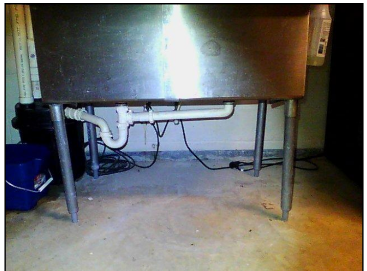
132. Laundry Area: No issues
