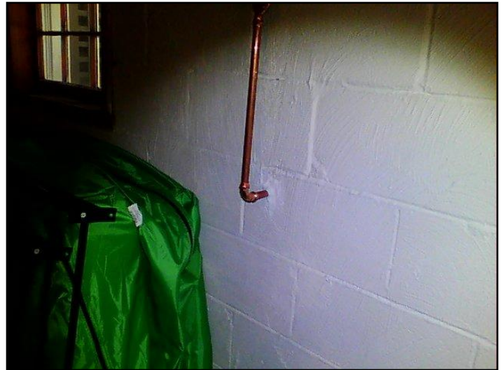
122. Plumbing Fixture/Penetration: No issues
