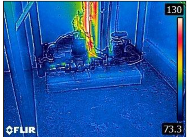
100. Plumbing Fixture/Penetration: No issues
