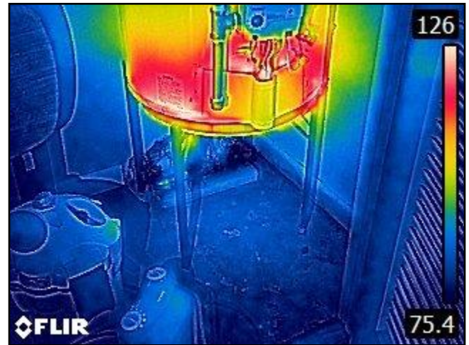
98. Plumbing Fixture/Penetration: No issues
