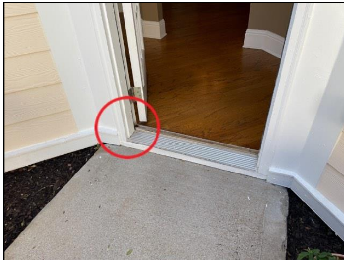
14. Rot/Insect damage
