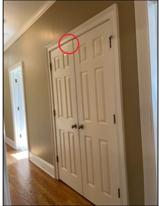
62. Does Not Latch Properly - Click for DIY Video
