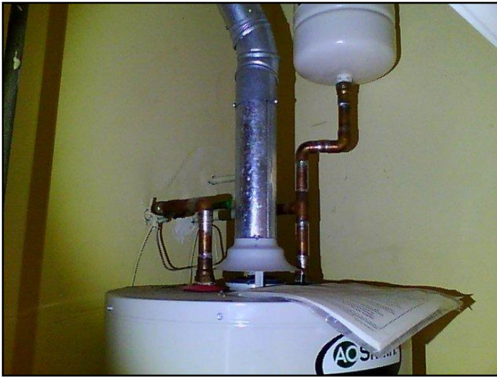
95. Plumbing Fixture/Penetration: No issues
