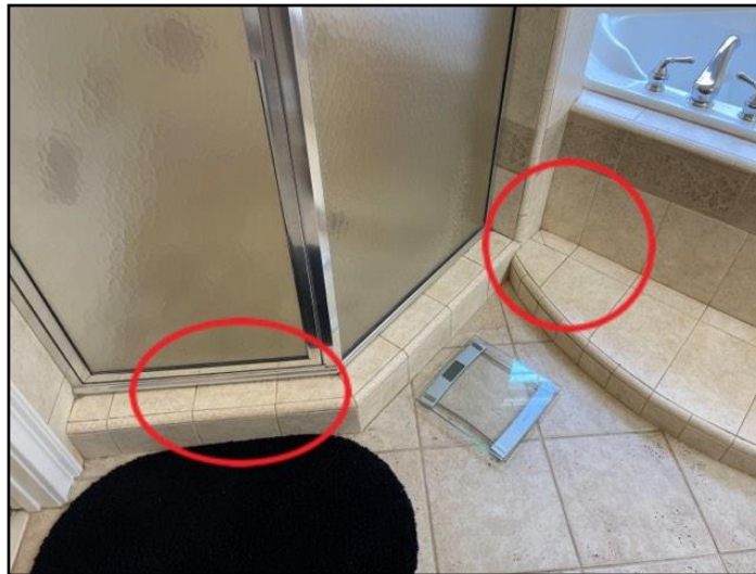
46. Loose/cracked tile
