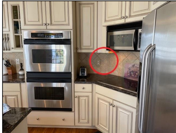
23. Loose Receptacles (Outlets) noted
