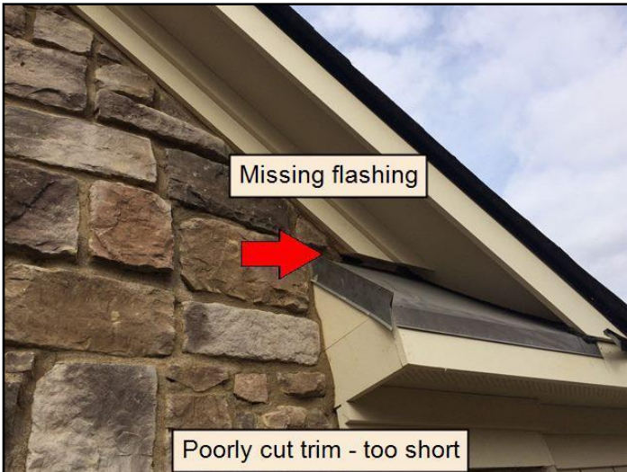
5. Flashings incomplete or ineffective
