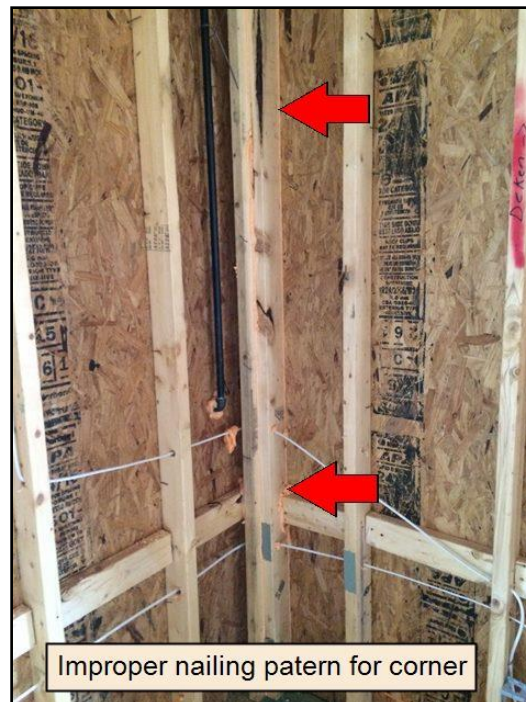
29. Poor nailing
