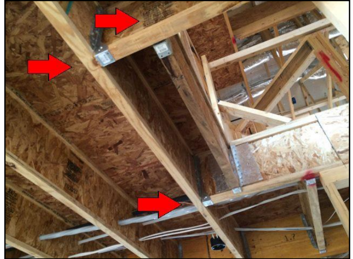
19. Poor end bearing, joist hanger connections
