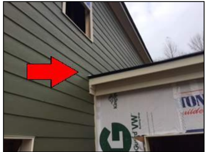
3. Flashings missing
