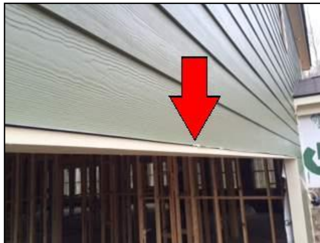
7. Flashings incomplete or ineffective
