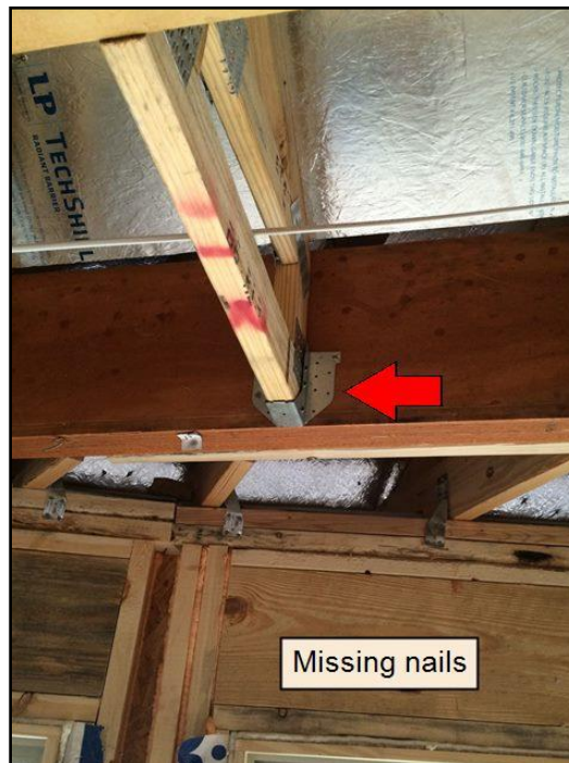
14. Poor end bearing, joist hanger connections
