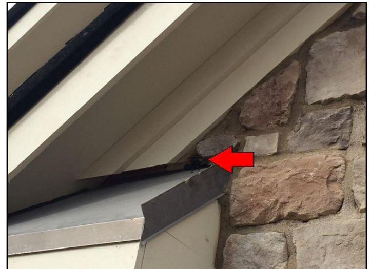
6. Flashings incomplete or ineffective
