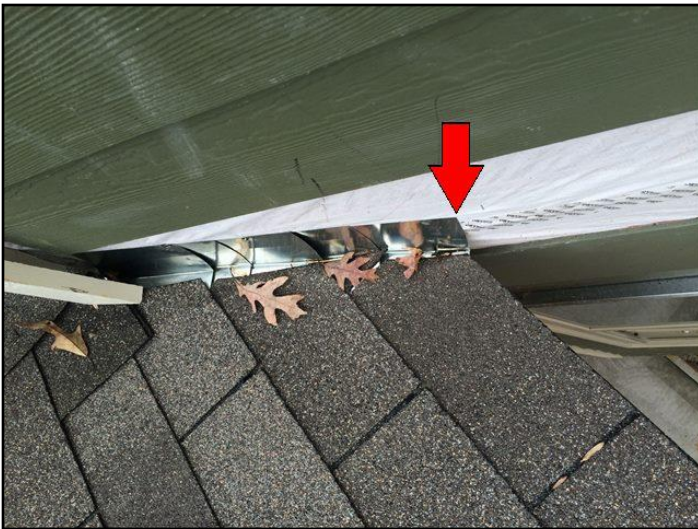
2. Flashings missing
